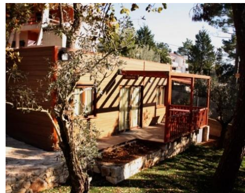
Figure 27 – Caves Houses (bungalows)
